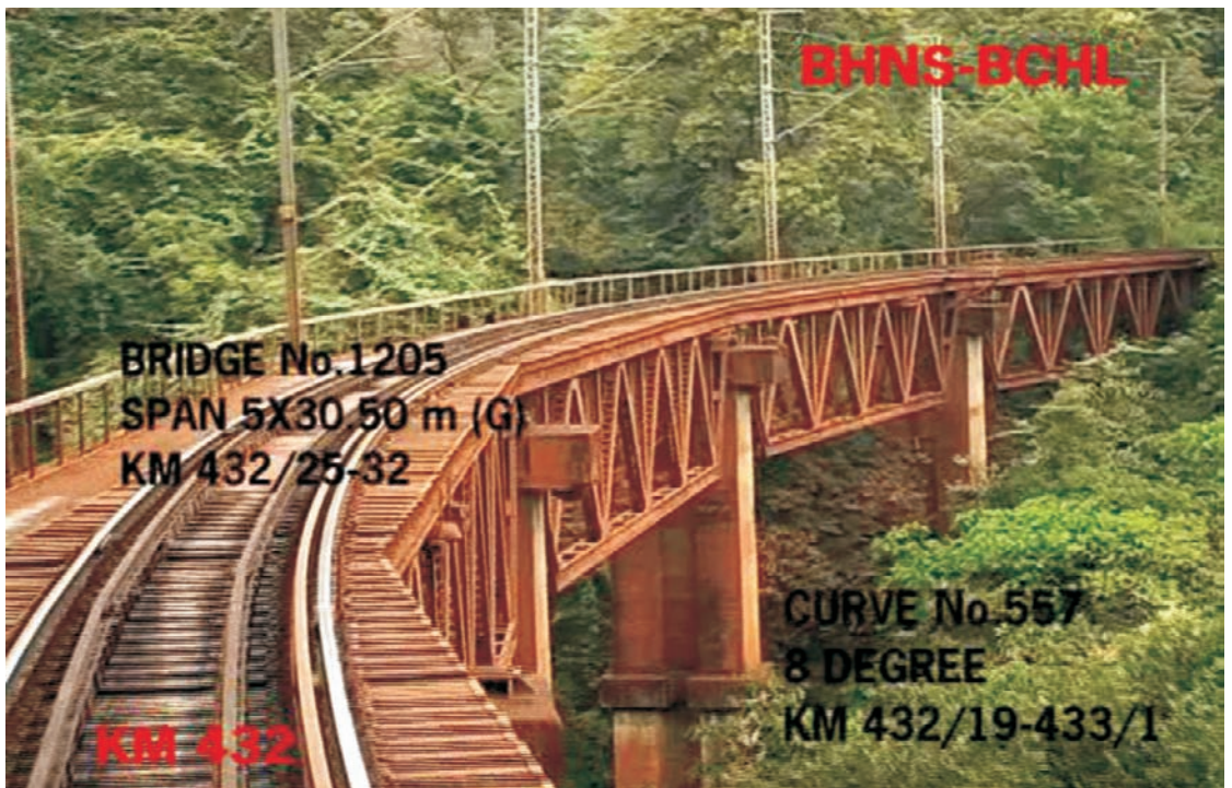
(d) Nerli Gorge Bridge (No. 1298; 5×30.48 M under slung girders on 8 curve) at km 432/25-32 in Bhansi – Bacheli Section
