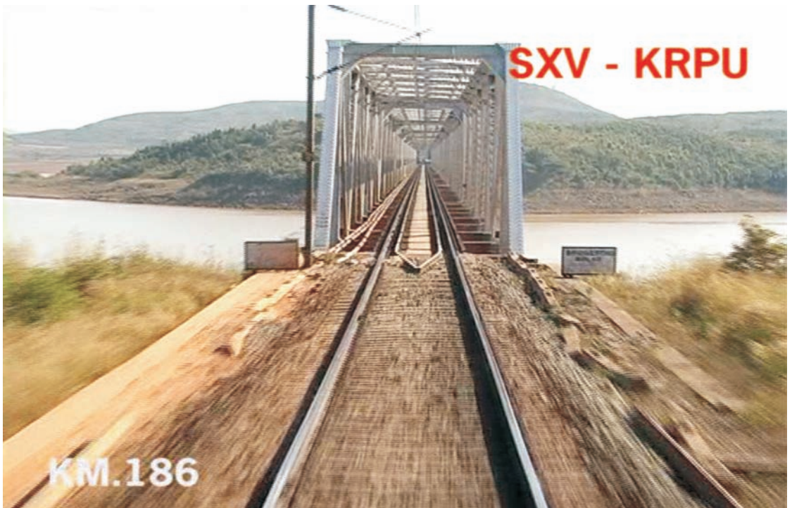
(b) Kolab Bridge (No. 413; Span 10 \times 45.72\text{m} ) at km 186/4-16 in Suku-Koraput Section
